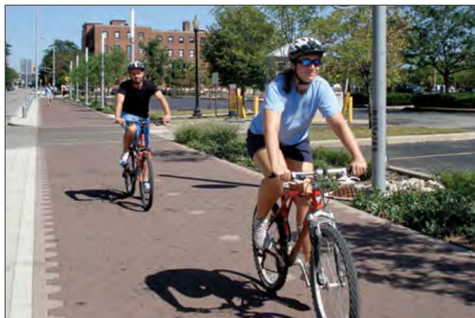
A Cycle Track provides one bicycle lane in each direction and can be separated from adjacent vehicular traffic by bollards.
