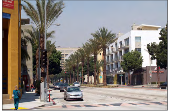
Multi-colored concrete sidewalks provide a colorful path for pedestrians to cross a relatively wide arterial street.
