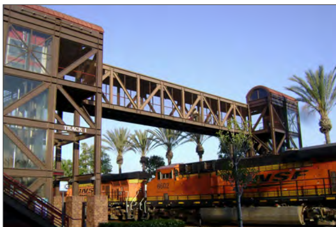
Example of a pedestrian bridge over railroad tracks.
