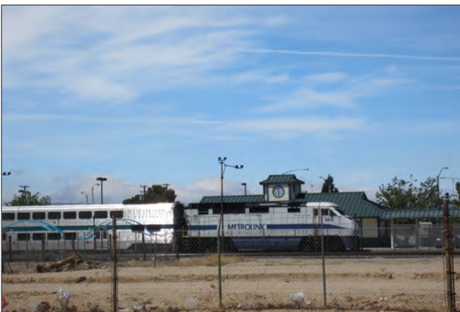
A Metrolink Train at the Lancaster Station
