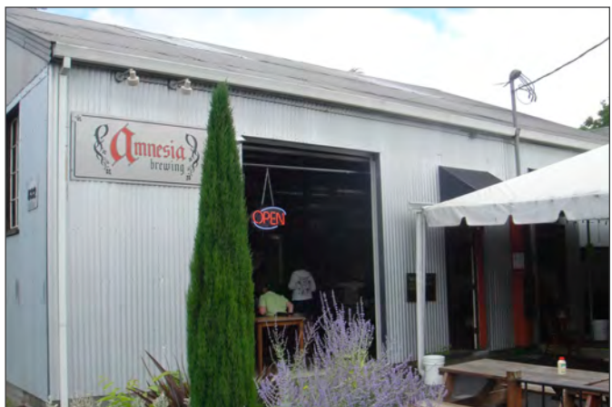
Industrial building adapted for a retail business.
