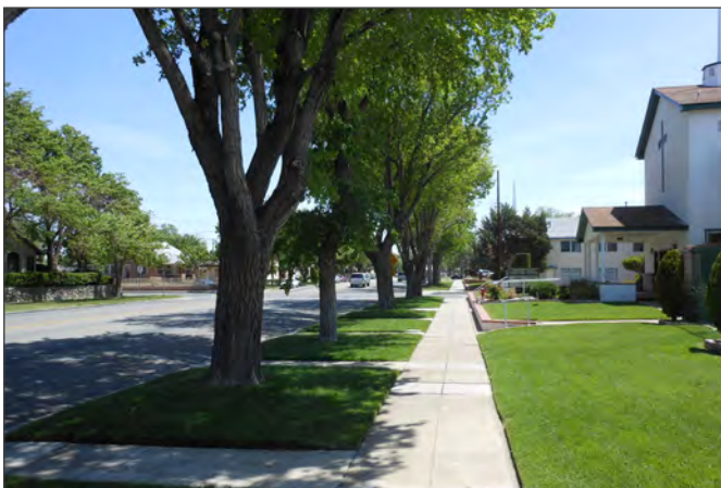
Beautiful streetscape along Lancaster Boulevard, looking east from Trevor Avenue, provides a model for some new STVPA streets.
