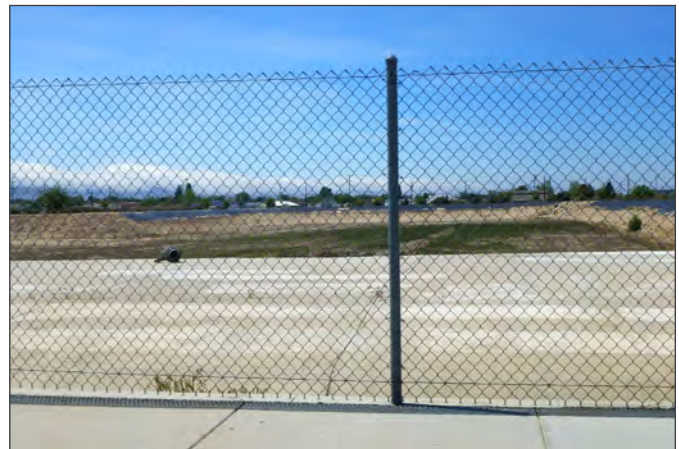
View of the stormwater detention basin from Division Street.
