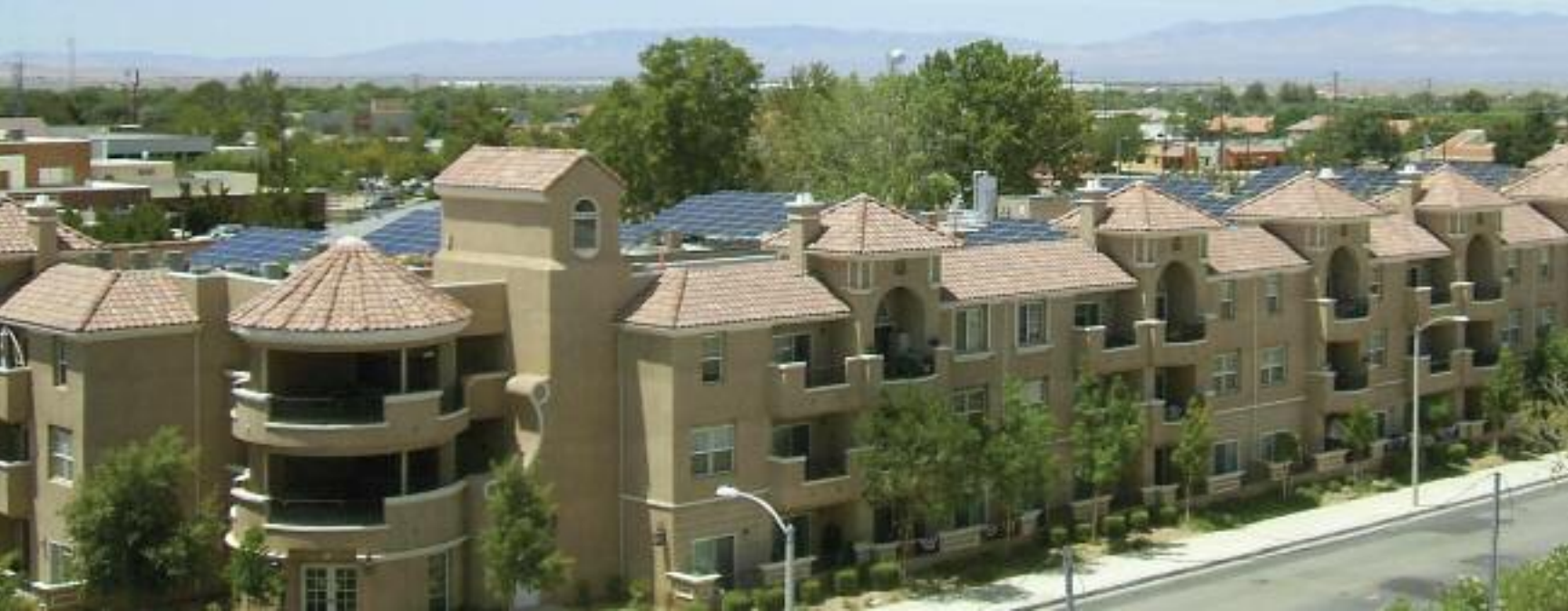
SolarCity roof installation at Arbor Gardens in Lancaster, CA
