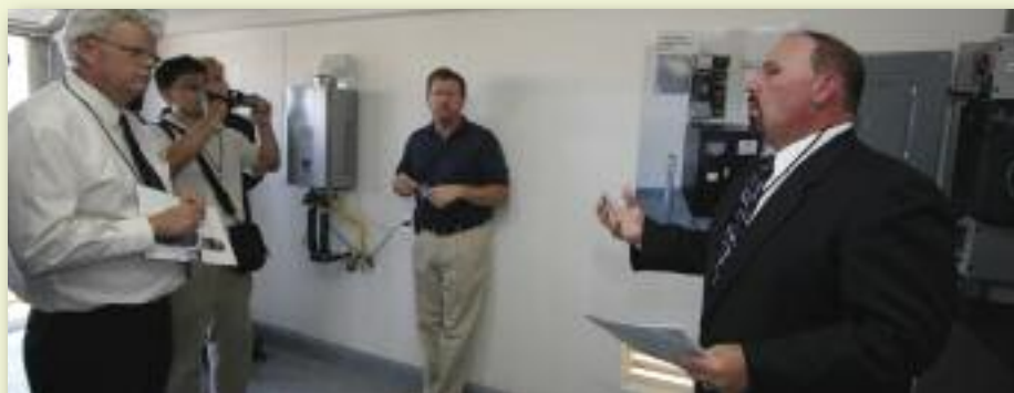
Thomas DiPrima of KB Home explains the components of future home electrical systems, including a solar inverter and lithium battery pack.
