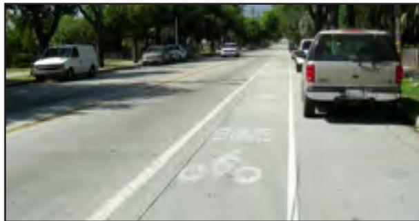
Figure 12-3: Bike Lane Striping and Stencil
