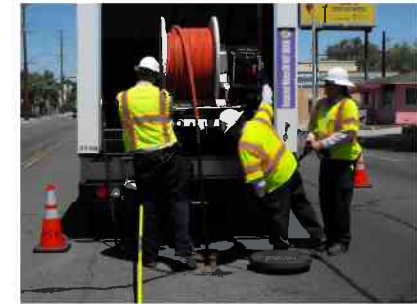
Preparing for pipe cleaning with hydro-jetting
