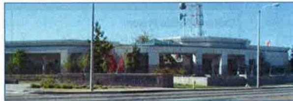
Figure 14: LASD Lancaster Station
