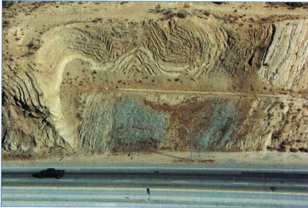
Figure 27: Palmdale Road Cut
