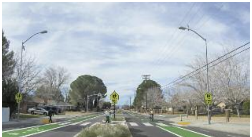
Enhanced crossing with the pedestrian refuge island and rapid flashing beacons.
