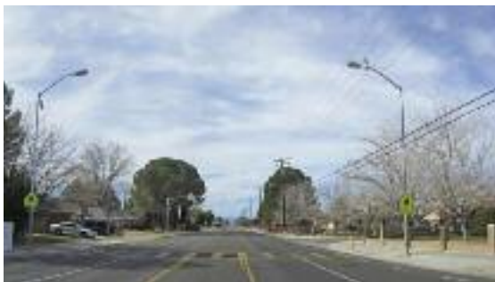
Existing school crossing on Lancaster Boulevard at 12th Street West.
