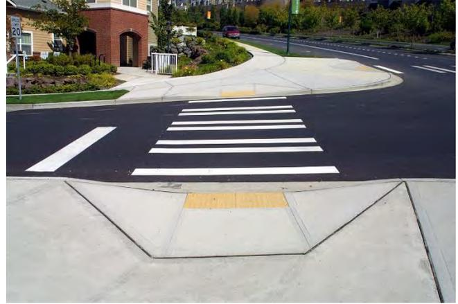
*Curb ramps should include a level landing pad.*
