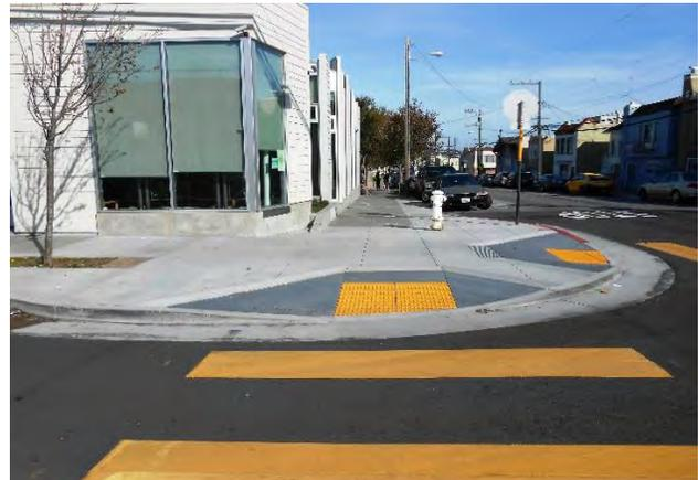
*Unidirectional ramps can be installed in conjunction with a corner bulbout at intersections.*
