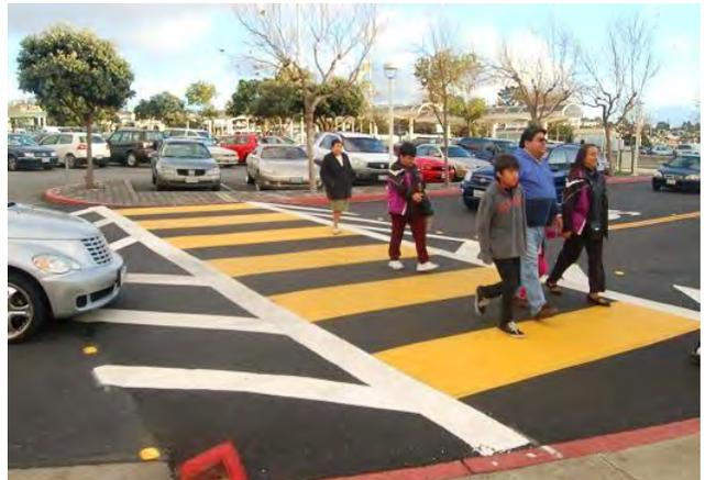
*Raised crosswalks should be wide enough that both the front and rear wheels of a passenger vehicle can sit atop the speed table.*
