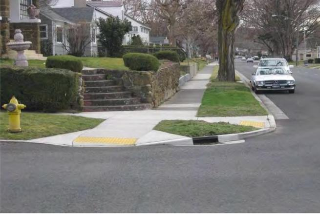
*Curb ramps should be accompanied by detectable warning strips.*
