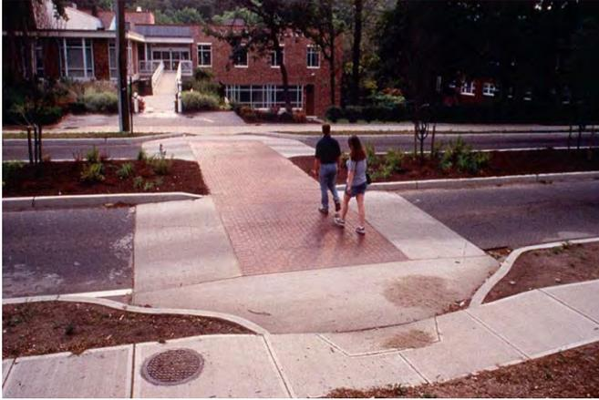
*Raised crossing should not impede street drainage patterns.*
