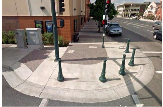
*Corner bulbouts should extend the full width of a parking lane*
