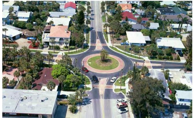
*Roundabout design should reduce relative speeds by requiring vehicles to negotiate the roundabout along a curved path.*
