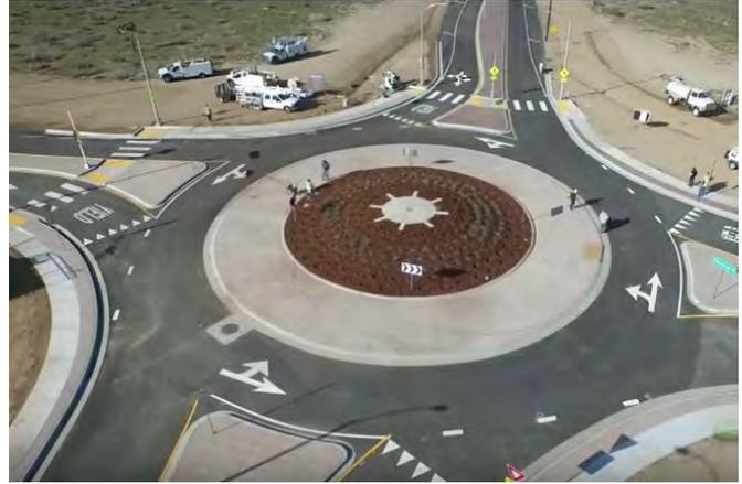
*At single lane roundabouts, the pedestrian crossing should be at least one vehicle length from the yield line.*
