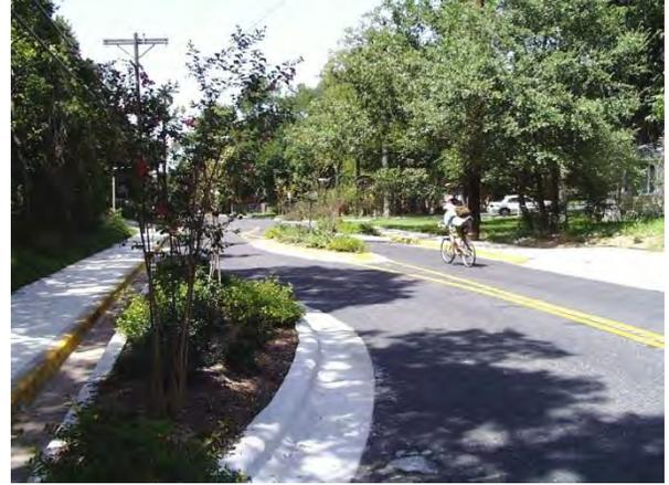
*Typically consist of a set of 2 or 3 curb extensions set in an alternating pattern.*
