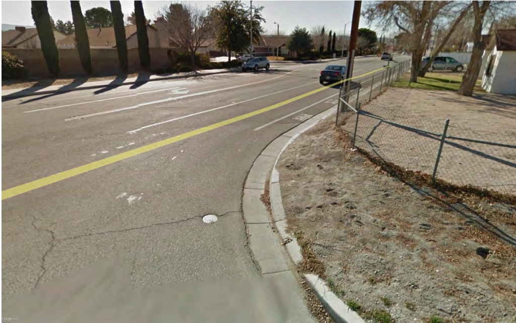
Figure 1- Typical Conditions in the Urban Core. Sidewalk Gaps Cause Pedestrians to Walk Close to Vehicular Travel Lanes
