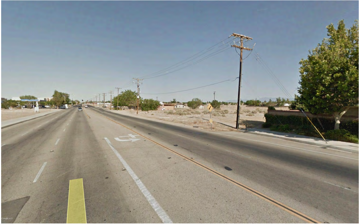
Picture 11 - Avenue I, 7th Street East to Challenger Way. No Sidewalk, Curb and Gutter
