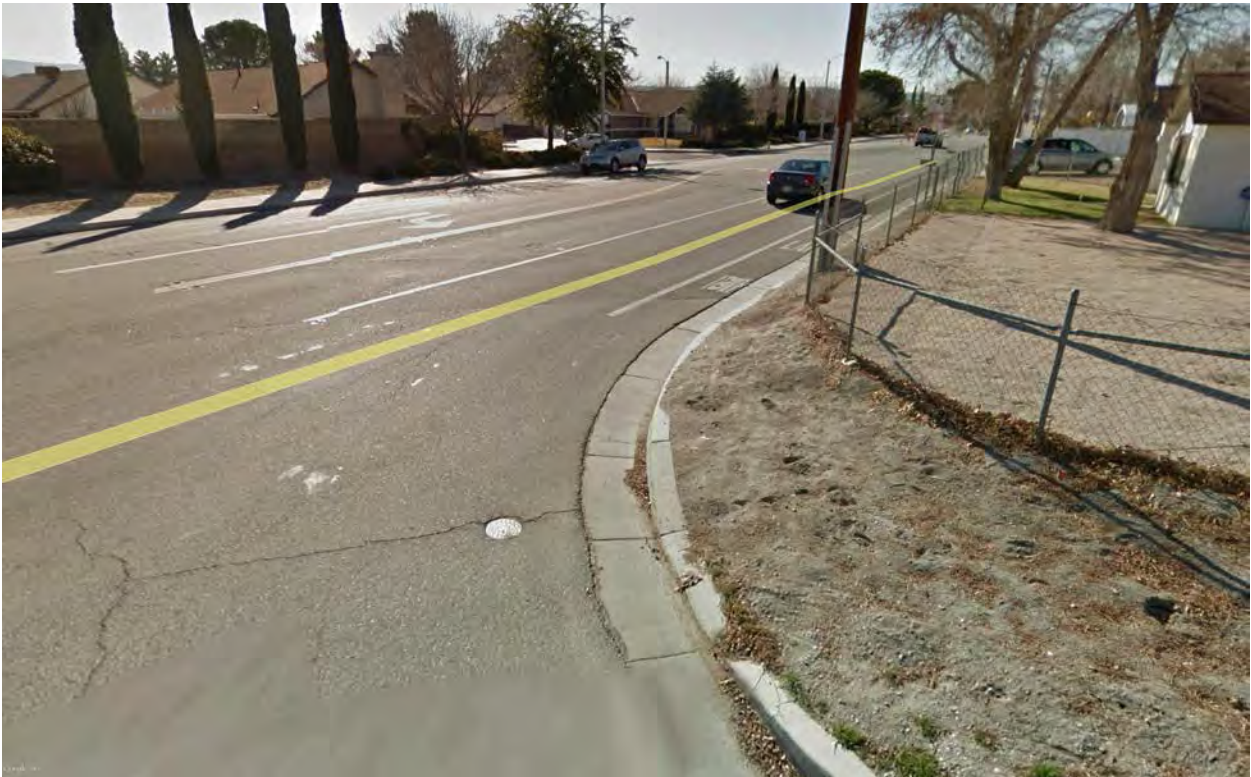
Picture 18- Avenue K-8, 20th Street West to 18th Street West. North Side Has No Sidewalk and Not Enough Room for Pedestrians.
