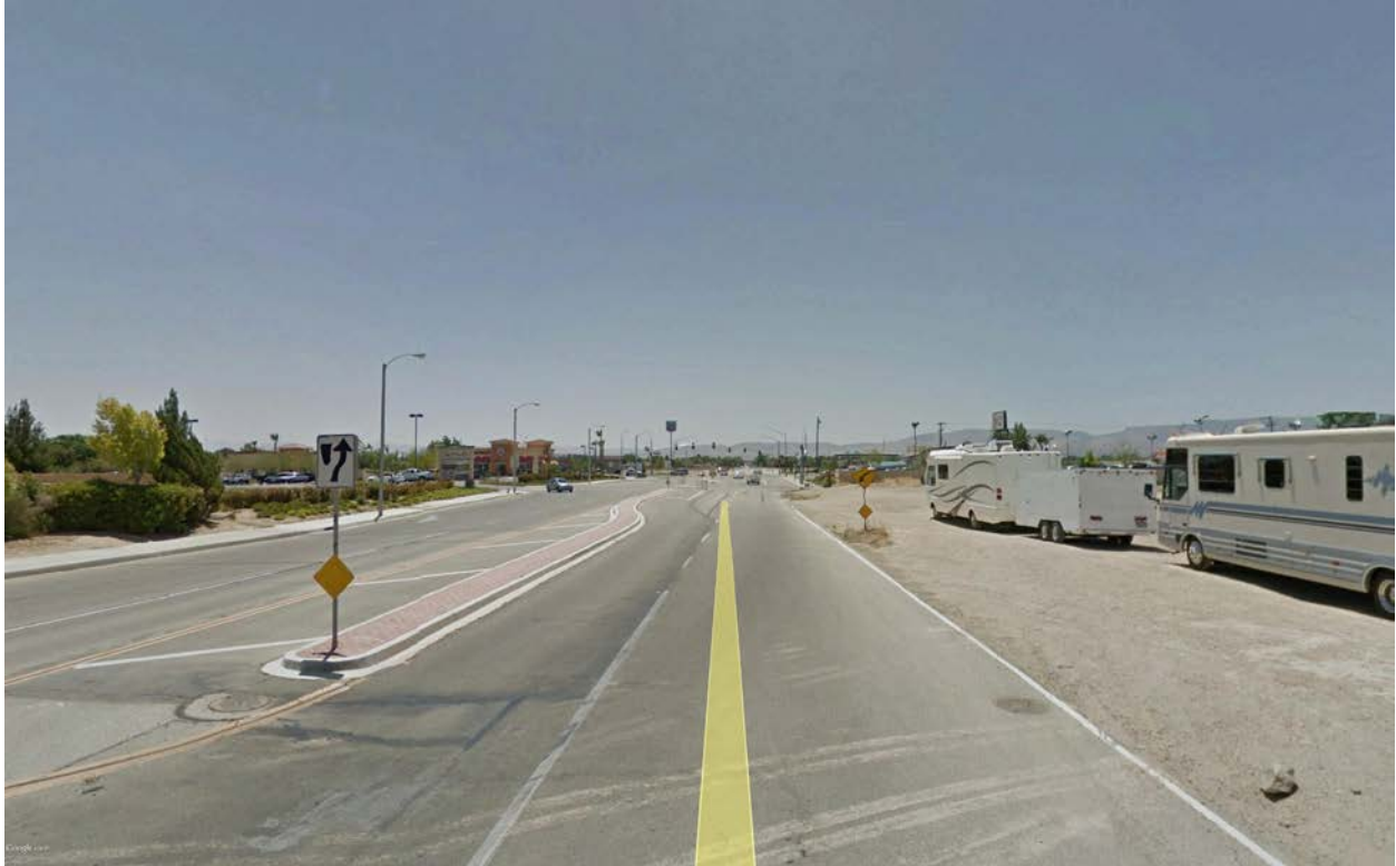
Picture 23 - 20th Street West, Arbuckle Way to Avenue I. No Sidewalk
