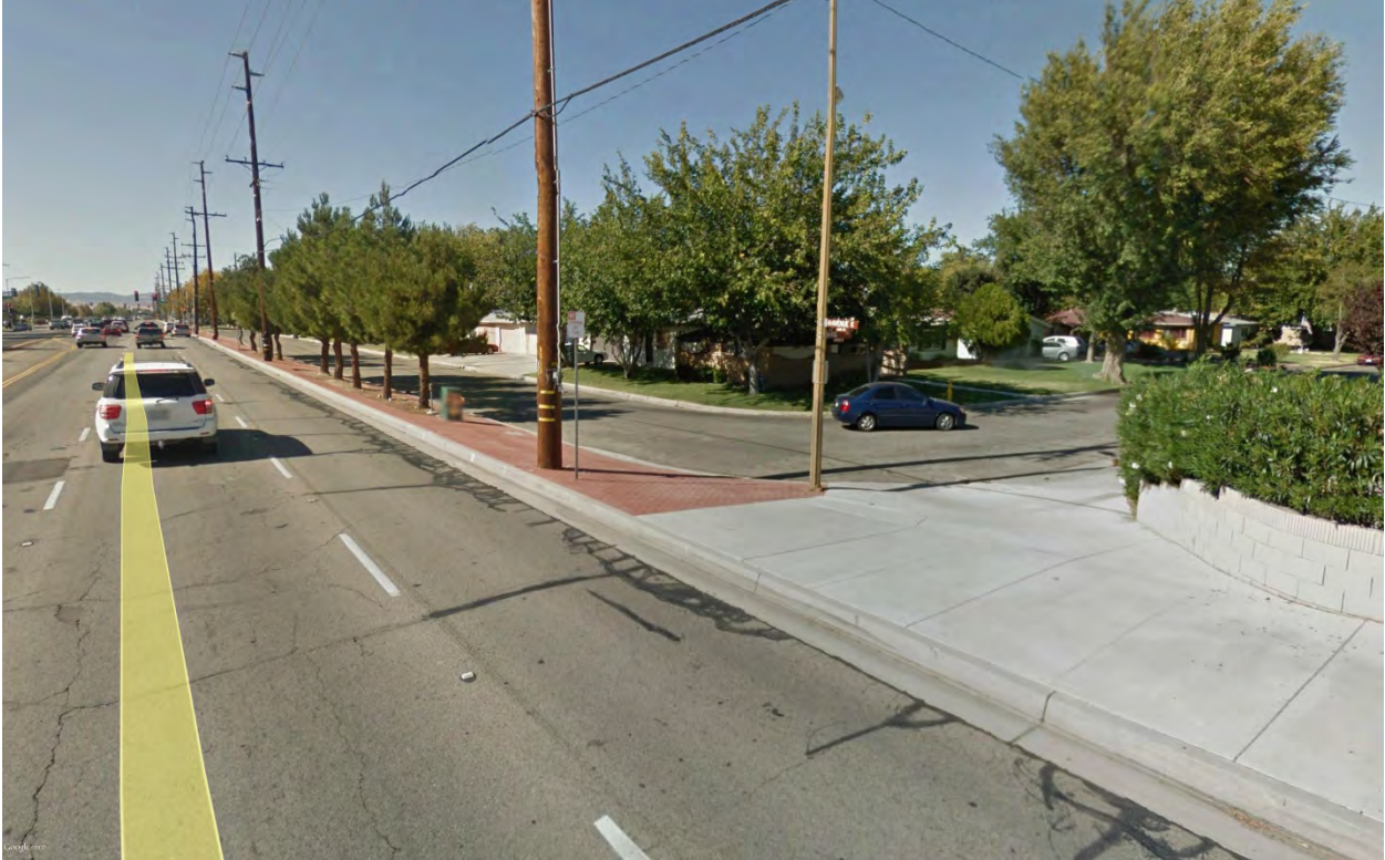
Picture 17 - Avenue K, Gadsden Avenue to Park Avenue. No Sidewalk on the North Side, Pedestrians Have to Walk on the Frontage Divider
