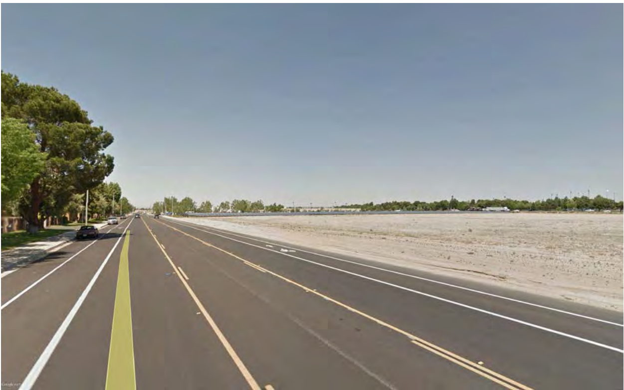
Picture 26 - 15th Street West, Park Somerset Drive to Avenue L. No Curb, Gutter and Sidewalk
