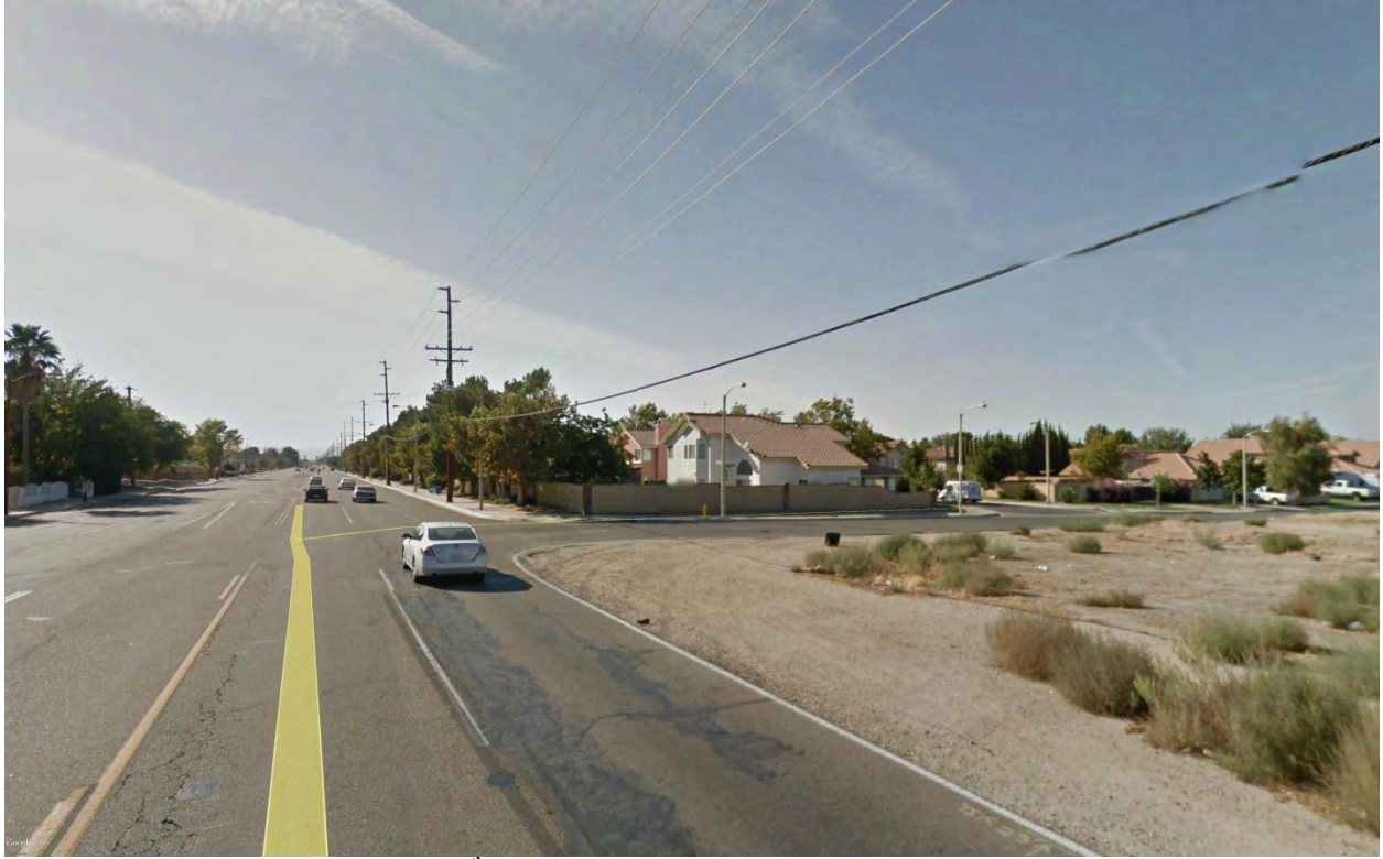
Picture 5 - Avenue K, 7th Street East to 8 th Street East. No Sidewalk, Curb and Gutter
