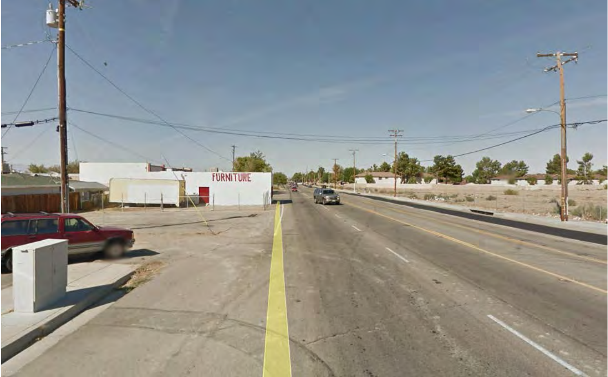
Picture 31 - Division Street, Kettering Street to Avenue J. No Sidewalk, Curb and Gutter. Pedestrians Have to Walk Close to Traffic Lanes
