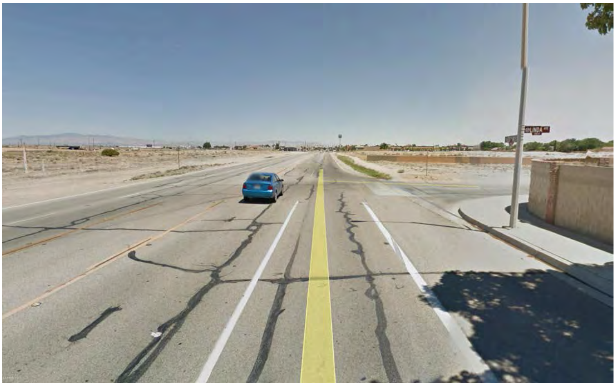
Picture 24 - 20th Street West, Avenue I to Louise Avenue. No Sidewalk, Curb and Gutter on Both Sides Leading to Commercial Area
