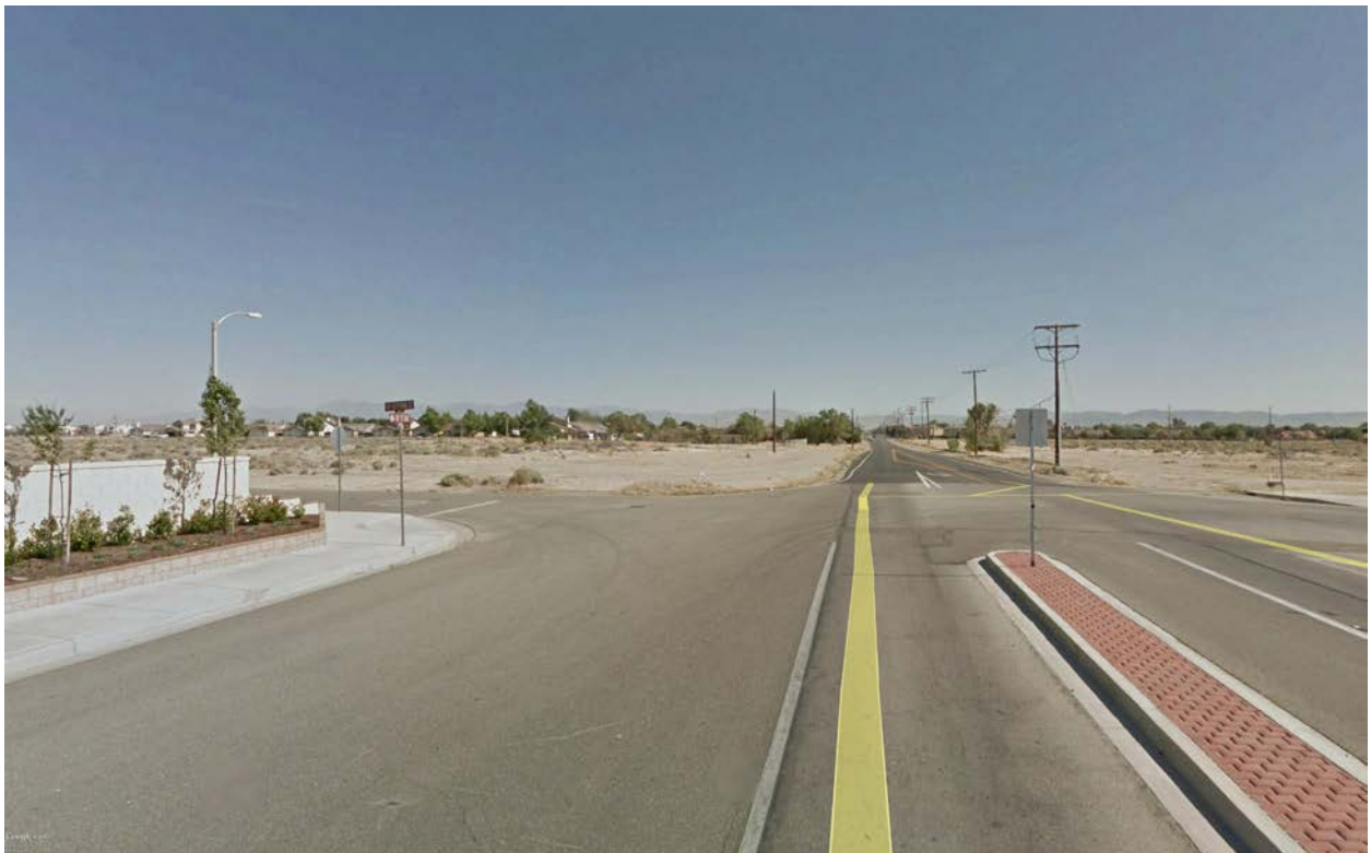
Picture 36 - 20th Street East, Jackman Street to Lancaster Blvd. Gaps in the Sidewalk
