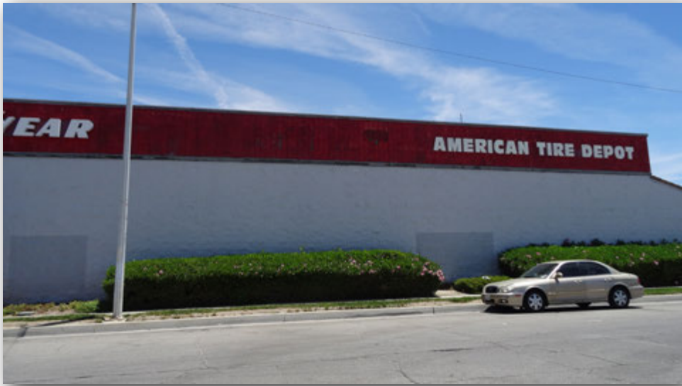
View Looking East
