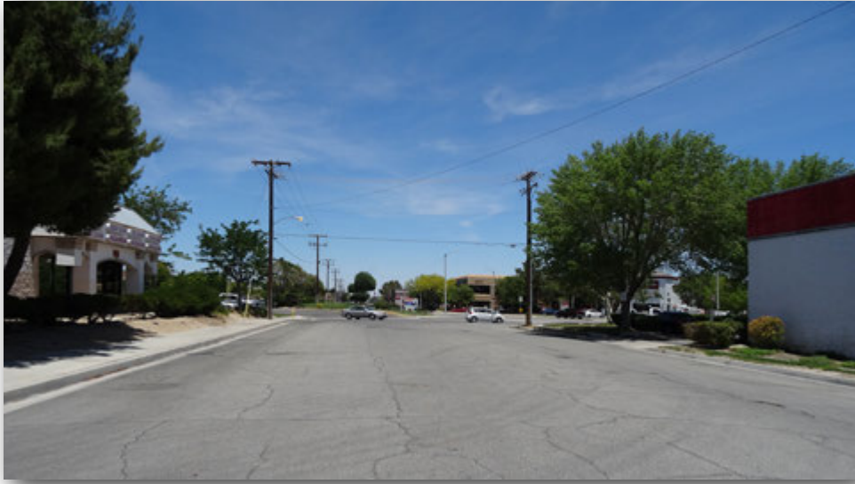
View Looking North
