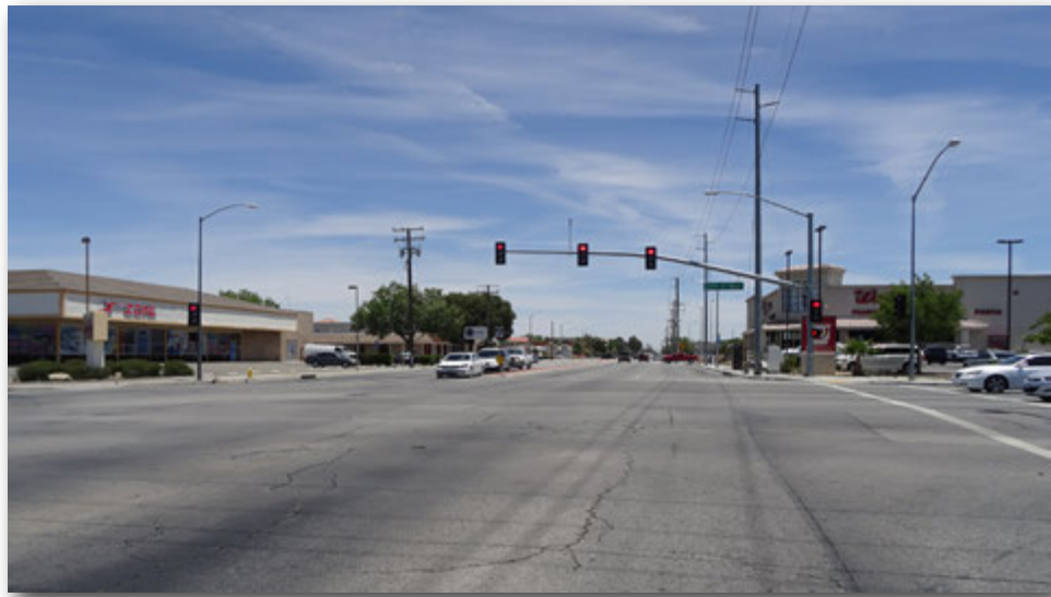
View Looking East
