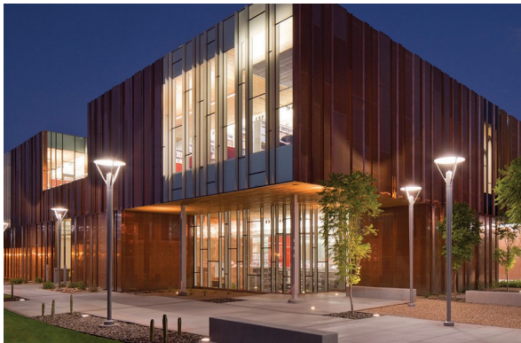
Indirect LED post-top luminaires may be suitable for parks and public spaces.
