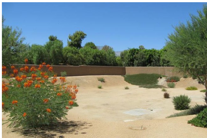
Stormwater detention areas help manage runoff from rain events.
