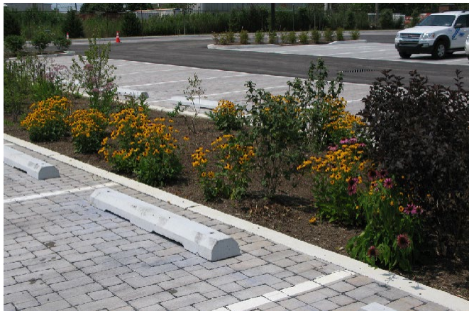
Parking with permeable pavers and rainwater collecting planters.
