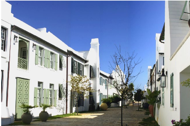
A paseo with flagstone and embedded planters that receive runoff.
