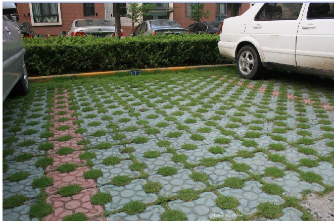
Permeable pavers within a parking area.
