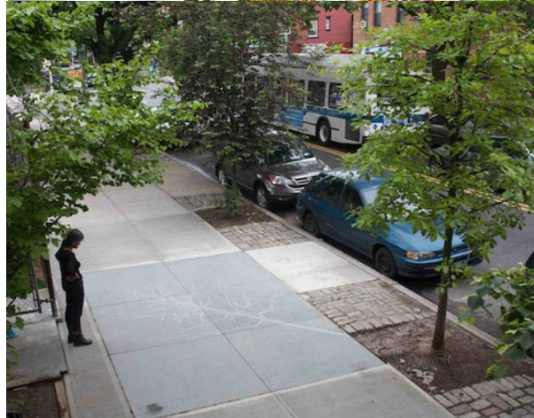
For streets lined with a mixture of office, retail, and residential parkways may be filled in with permeable pavers to increase sidewalk space.
