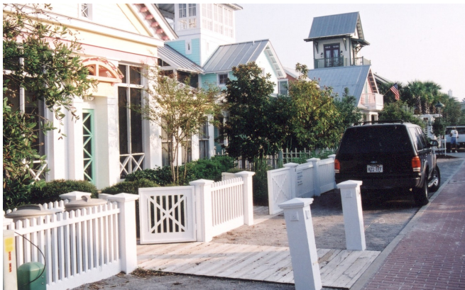
Permeable materials such as pavers, decomposed granite, or gravel can be applied to parking lanes in a variety of settings.
