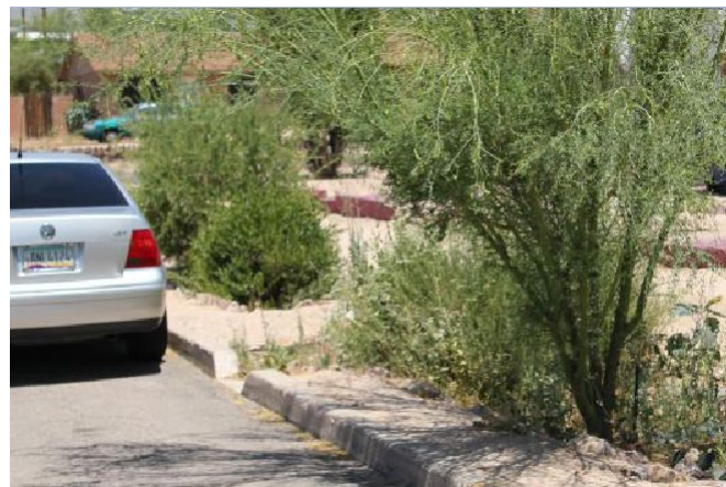
Drainage channels may be cut into street curbface to allow street run-off water to drain into medians.
