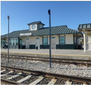
Lancaster Metrolink Station
