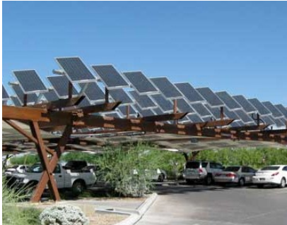
Sustainable design in the form of solar and shade structures protecting a surface parking lot.
