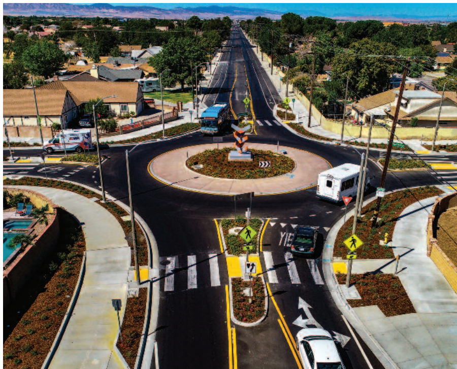
The City's latest roundabout, located at 15th Street West and Lancaster Boulevard, was completed in September 2019.
