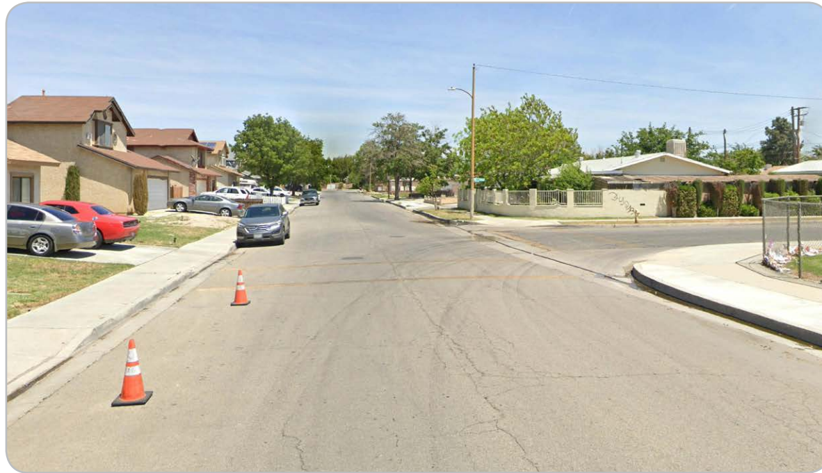
Kettering Street & Rodin Avenue Eastbound Lack of high visibility crosswalks, stop signs, and stop lines.
