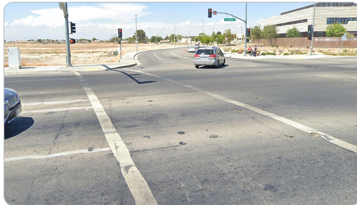
Avenue I & 3rd Street East eastbound Lack of high visibility crosswalks and advance yield lines.
