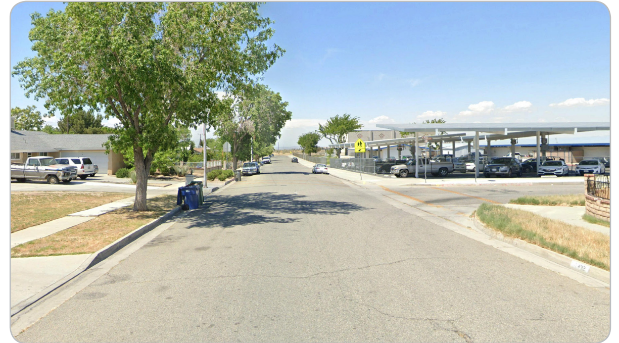
Avenue H11 & Foxton Avenue northbound Lack of high visibility crosswalks, stop sign, stop line, advance yield lines.
