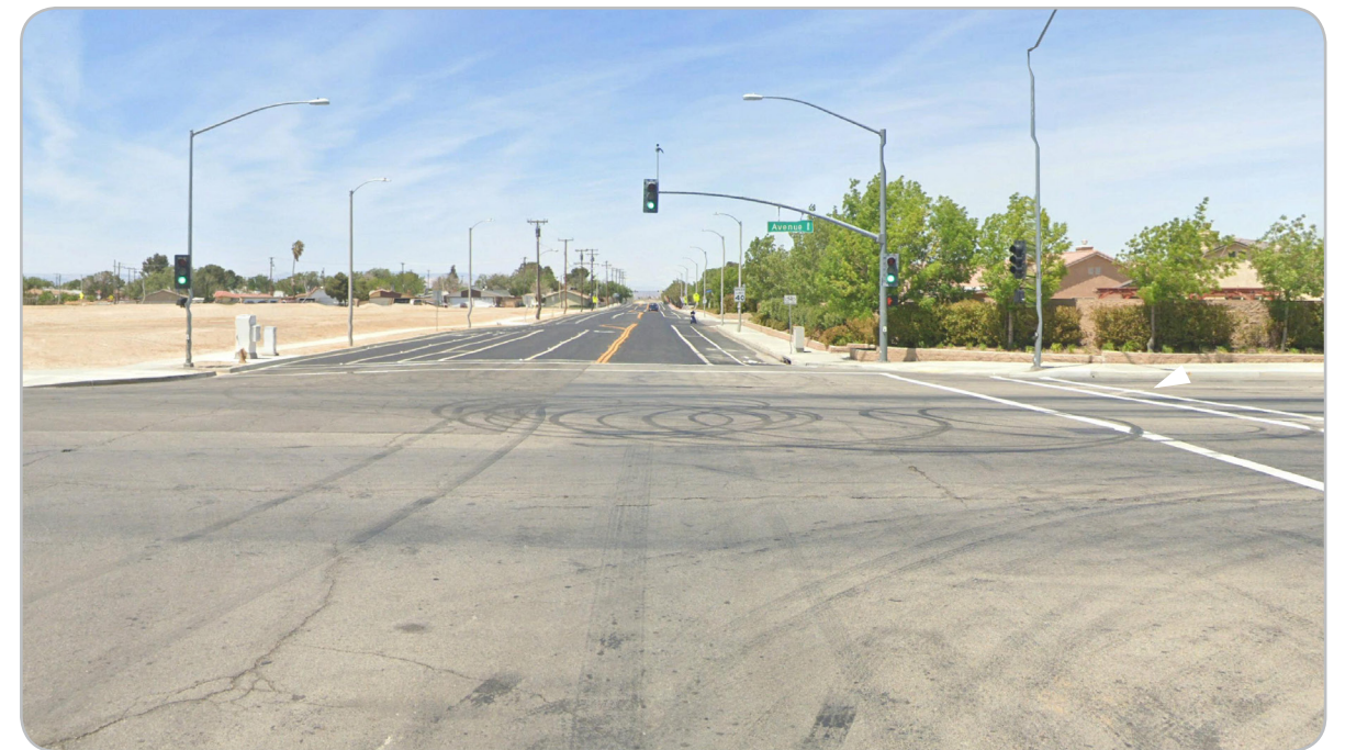
Avenue I & 5th Street East northbound Lack of high visibility crosswalks and advance yield lines.
