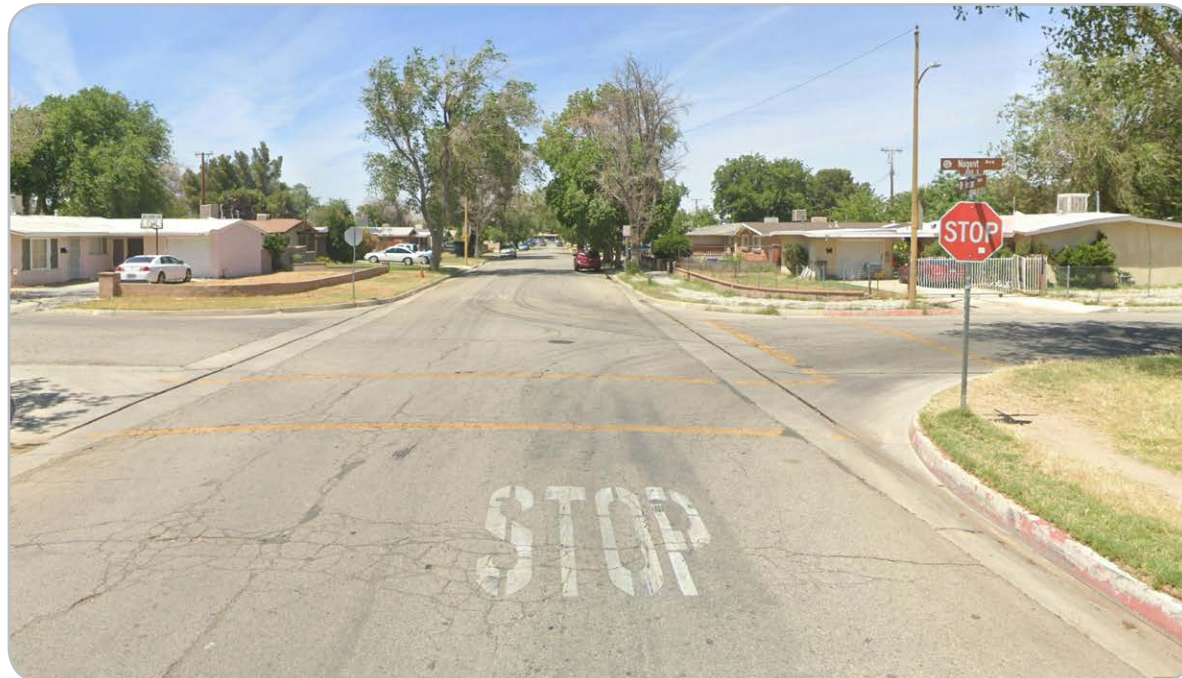
Nugent Street & Foxton Avenue northbound Lack of high visibility crosswalks, advance yield lines, stop lines, and sidewalk.
