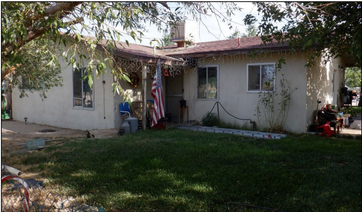
Photo 6: Building 1 (residence), June 17, 2022 (view north).
