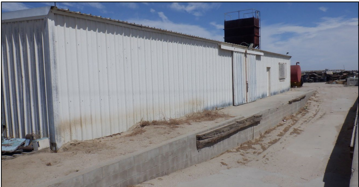
Photo 11: Building 6 (storage building), June 17, 2022 (view northwest).
