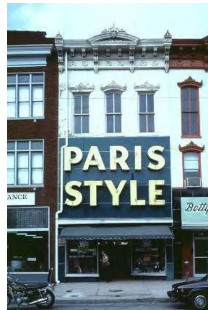
Inappropriate use of signage on facades:
