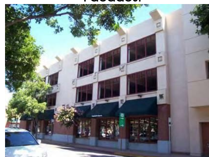
Examples of Appropriately Designed Parking Structure Facades:
