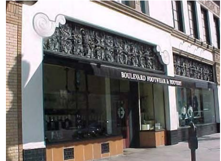
Awning and Marquee Signs:
