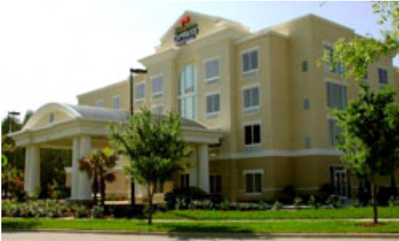
•Identifiable building entrance
