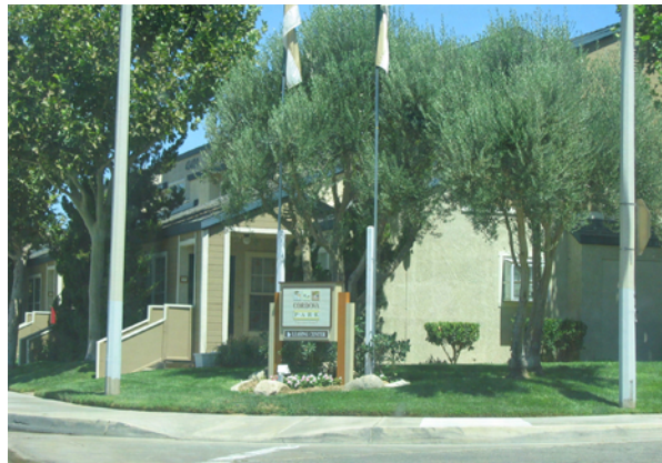
Apartment Complex North of Site
