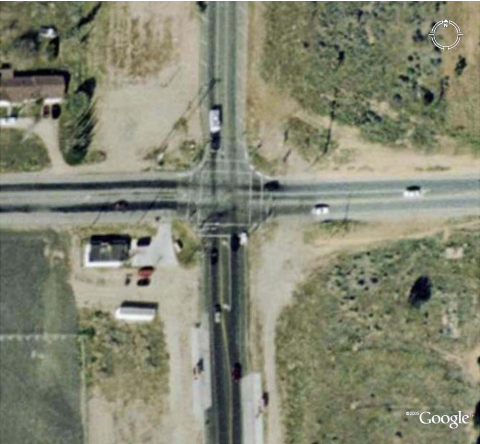
Ave L and 50th St
