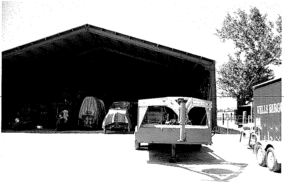
Photograph No. 8: Storage barn, looking south, located on the southern end of the developed ranch area.
