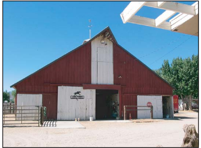
View 2: View of the barn. Note the steep gable roof, board-and-batten façade and the oversized sliding doors.
