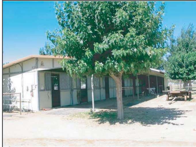
View 6: View of a service outbuilding.
