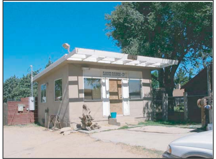
View 5: View of one of the service/office buildings of relatively modern construction. Note the unremarkable architectural character.
