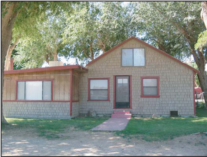
View 1: View of the small house. Note the shingled facade, non-original windows, and one-story addition.
