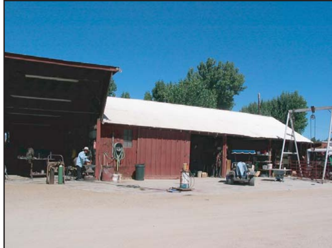
View 3: View of the shed. Note the features of the garage are similar to those of the barn.
