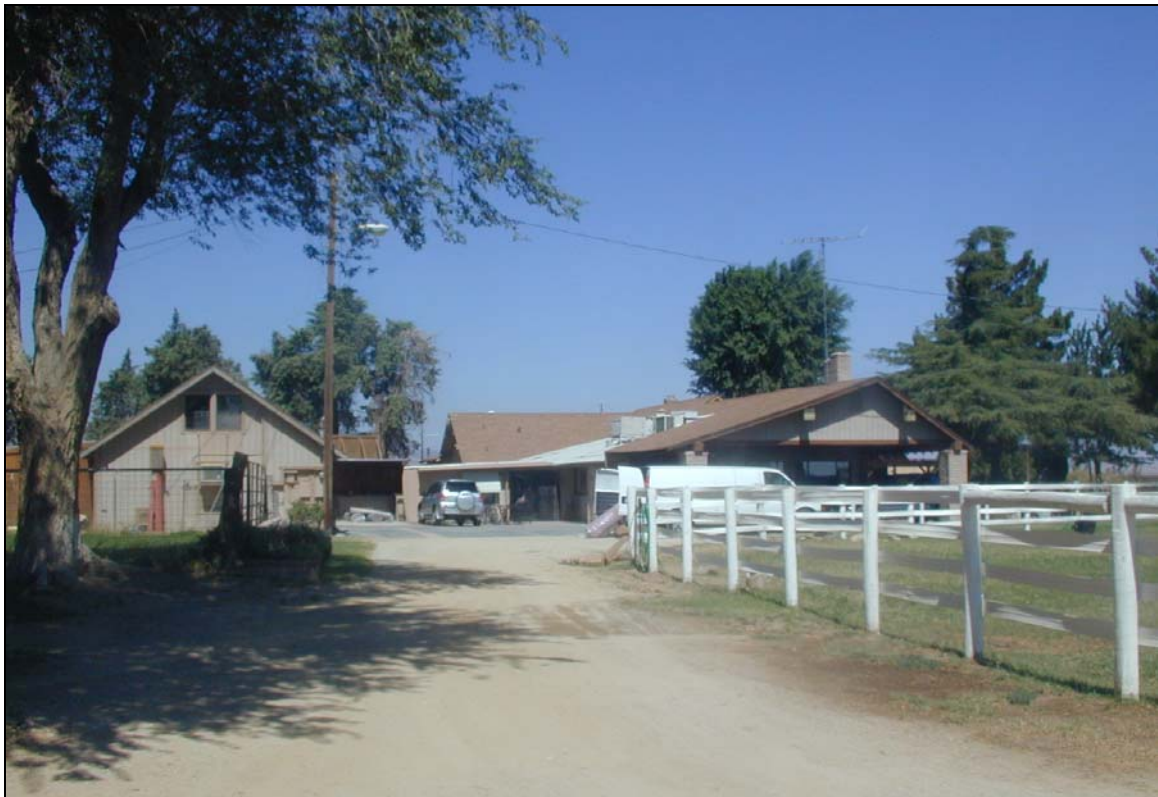
Figure 4-1 Lane Ranch residence, view to the west.
