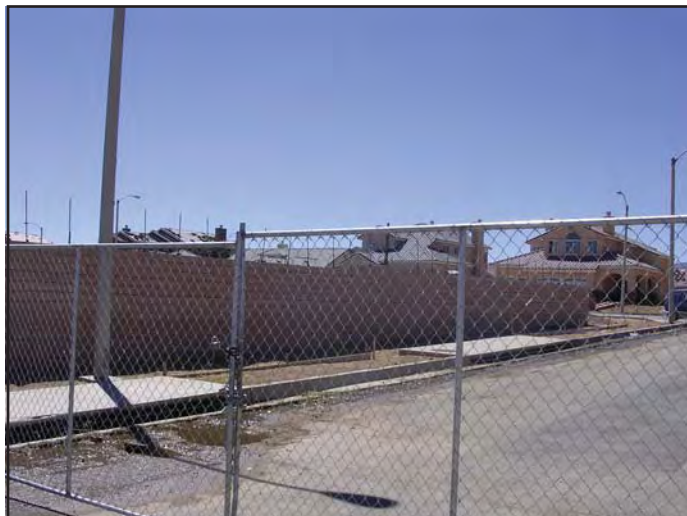
View 12: View of new construction east of project site from the corner of Avenue L and 57th Street West.
