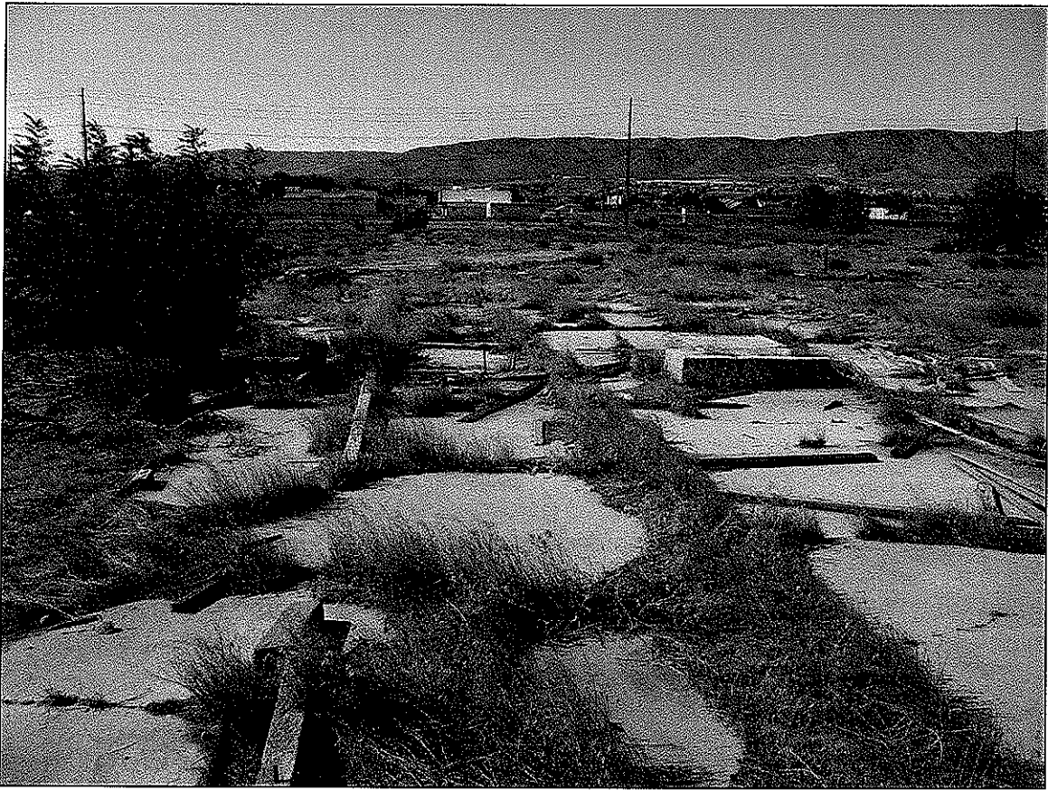
Figure 4-2 Concrete foundation in survey area, view to the south.
