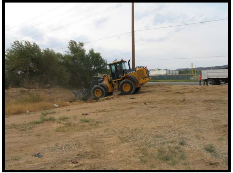
City of Lancaster clearing and re-grading off-site active drainage on July 10, 2007
