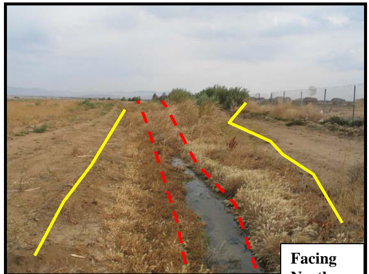
Offsite Active Constructed drainage, illustrating OHWM per Corps definition marked as the dashed lines and the top of banks per CDFG definition marked as a solid line includes the riparian vegetation.
