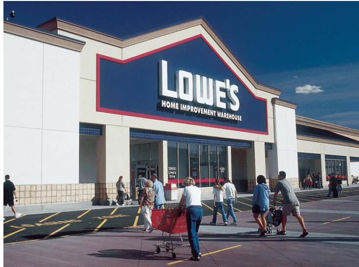
Located at the SEC of Ave. K and 10 th St West (Amargosa Project), this Lowe's was made possible through the Agency's ability to acquire and assemble parcels. Assembly of smaller parcels into larger, more marketable parcels is an important tool for economic development and job creation.
