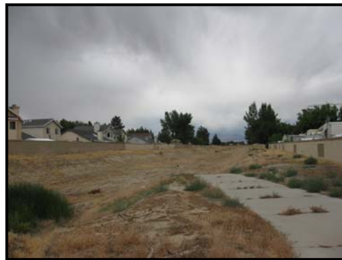
Lancaster Drainage Channel
